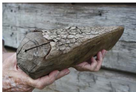
Closeup of a pine log wedge used as a supplemental means of chinking for the log structure.
