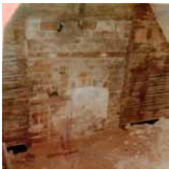
▲ Figure 3. Bricked in fireplace. Note stripped lathing and shadow of the original mantel.
